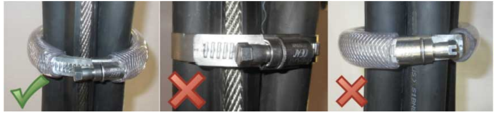
Fig. 27: Installation information for the cable clamps
