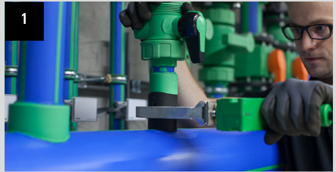
1. Welding-on of weld-on saddle set onto the main pipe
