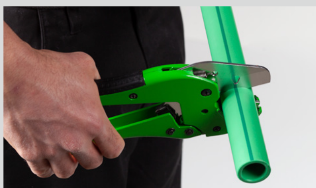
Cutting of the pipe
